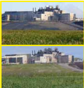
Reclamation of Slag Disposal Area: Aug 2006 (top) to July 2007 (bottom)
